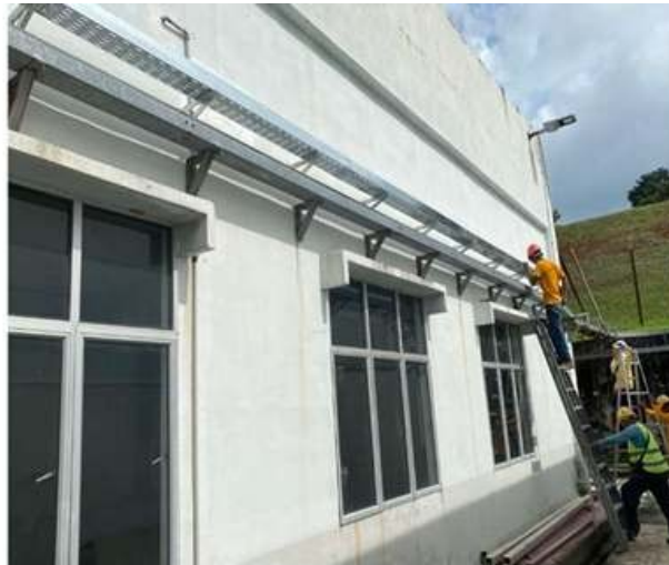
Installation bracket & cable tray from MSB room to G14 & G15
