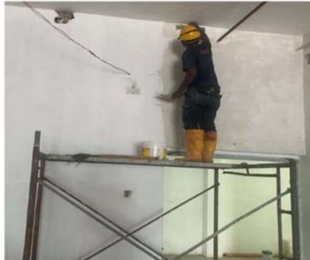
Skim internal wall inside G14 & G15 room
