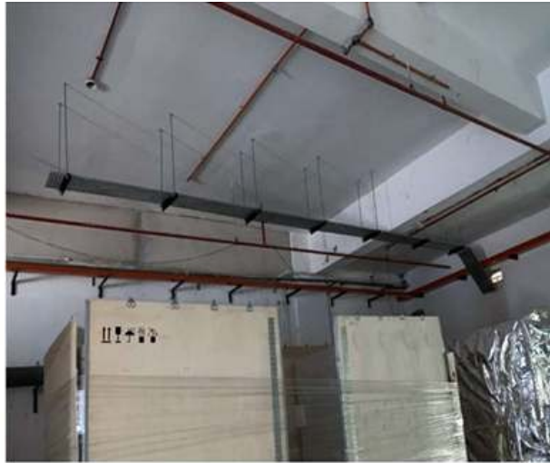
Installation bracket & cable tray from MSB room to G14 & G15
