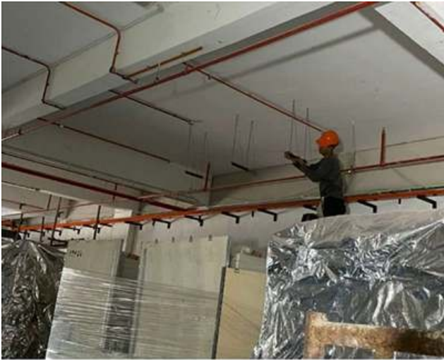
Installation bracket & cable tray from MSB room to G14 & G15
