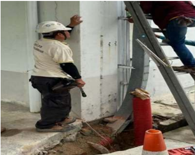
Installation bracket & cable tray from MSB room to G14 & G15
